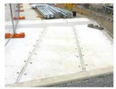
Slabs can be cut on site or in factory to suit exact dimensions
