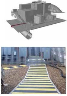
Alternate colours for high visibility in poor weather conditions
