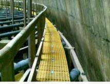
Standard Moulded FRP Grating Type 13 used as an anti-slip open mesh topping for existing structure
