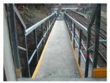
Service or temporary walkway access can be made safer with the use of Kite Safety Handrailing
