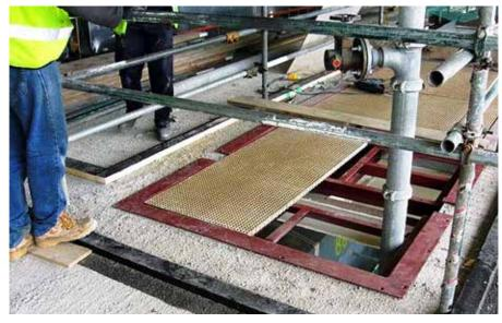
Top of lift shaft fitted with steel frames and fixed within a concrete slab and then decked with Mini Mesh FRP Grating Type 38 Lift Risers to prevent falls and loss of equipment tools during the build process and/or during routine maintenance
