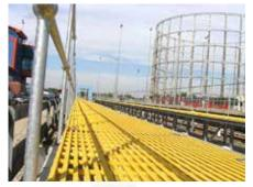
Pultruded FRP Grating Type 38 in hi visibility yellow providing maximum load capacity on wash bay platform in single direction
