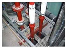
FRP Grating Lift Risers can be installed on each floor during the build to provide worker safety on-site; they can then be cut to suit permanent riser shaft equipment or services
