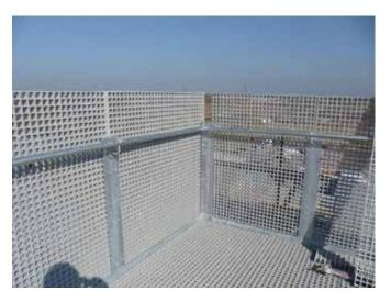
Open grid system ideal to screen items at height and to blend with walkway floor grating
