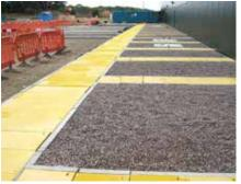
Pultruded through a die, Kite Slab exhibits an incredible strength to weight ratio producing a composite flooring structure that is rigid, strong, lightweight, non-corrosive, durable and maintenance free with an anti-slip surface.
